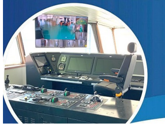
DP2 bridge control console
