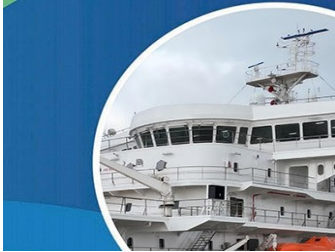
Bridge / accommodation block
