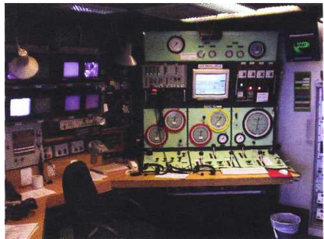
Figure 2.26 Dive Control Room
