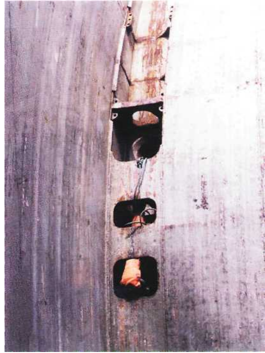
Figure 5.9 Deck Mounted Reel — Tie-in Arrangement
