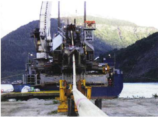
Figure 9.3 Pipe Lay Spooling
