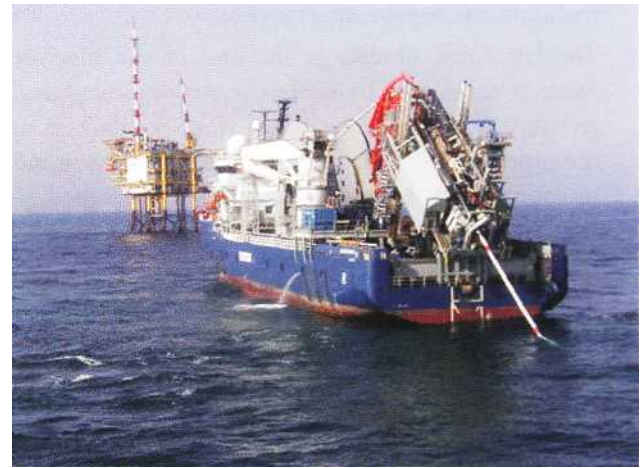
Figure 9-6 Pipe Lay Deployment Operations
