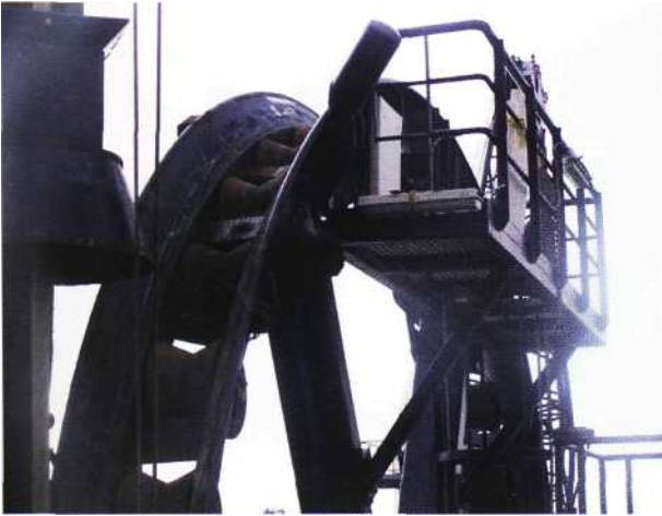
Figure 5.30 Vertical Lay System Tower — Upper Chute
