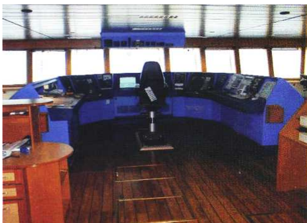
Figure 1.18 Subsea Viking - Forward Bridge Console for Navigation and Transit Control
