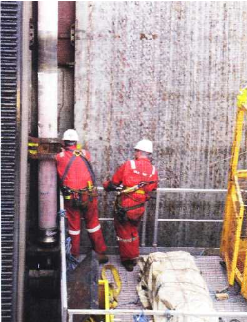
Figure 9.4 Pipe Lay Loading
