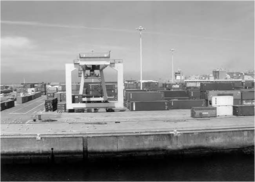
Fig. 8.31 Walkways, road paths and track rails for gantry cranes seen alongside the berth, opposite the terminal stacking gantries. Container avenues lying parallel to the ships berth.
