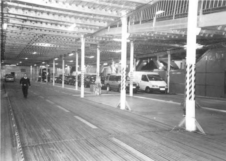
Fig. 7.14 Example vehicle deck of the enclosed cargo compartment of a high-speed passenger vehicle ferry operating in the Irish Sea region of the UK coastline. Steel pillars support aluminium upper decks and the internal, angled ramp is seen at the upper right-hand side of the view. The deck structures are manufactured in unpainted aluminium to save increased weight.
