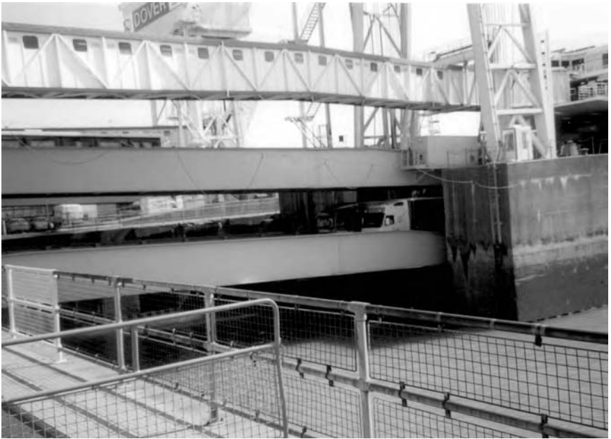
Fig. 7.23 An example of the ship-to-shore, shore-to-ship access 'link spans' which operate at the Dover Terminal. The upper enclosed passage is for passenger transit, while the lower open top links accommodate car and truck vehicle traffic.
