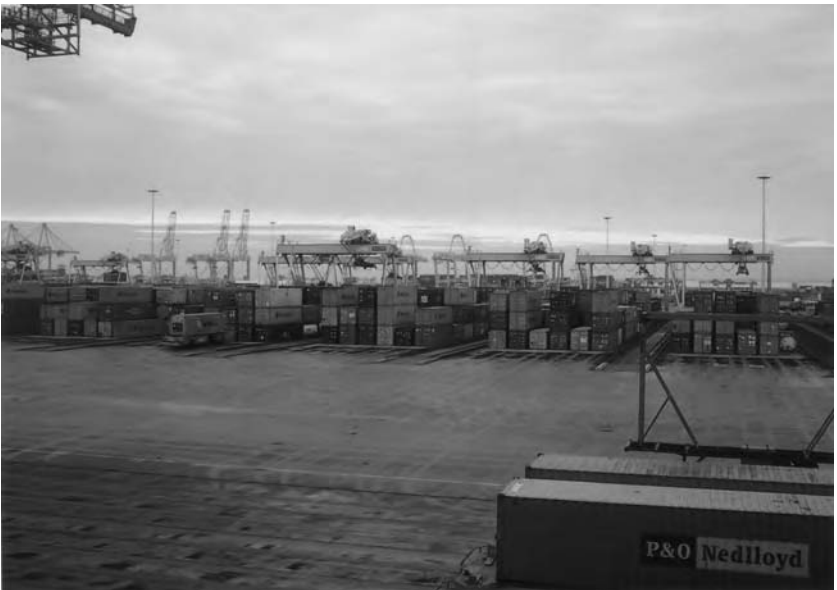
Fig. 8.28 Automated stacking cranes provide unit movements to the terminals container stack. The containers being loaded to driverless ground-handling transports.
