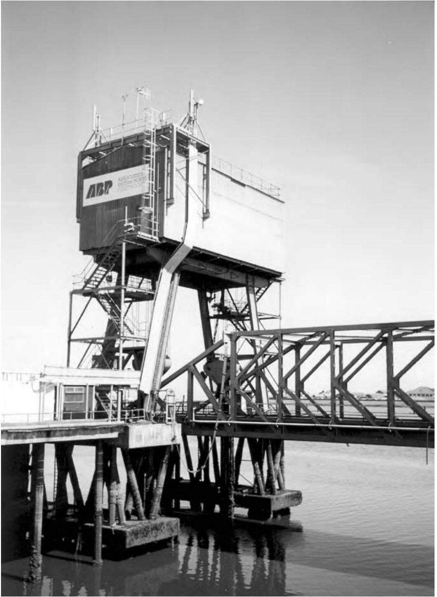
Fig. 7.24 Link span operation. A typical link span machinery housing for hoisting and lowering the link span down to a position above the waterline. The stern ramp of the Ro-Ro ferry then lowers her stern ramp onto the links driveway to permit discharge of vehicles. The rise and fall of tide of 10.5 m is countered by the adjustment of height to the link span to allow continuous operations no matter what state of tide.
