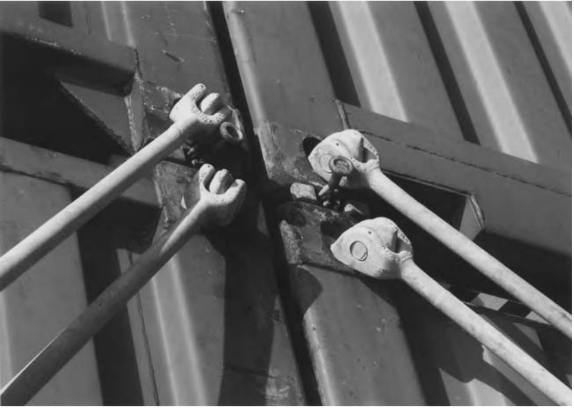
Fig. 8.22 Container lashing bars, seen secured from the main deck to the first and second tier of deck containers.
