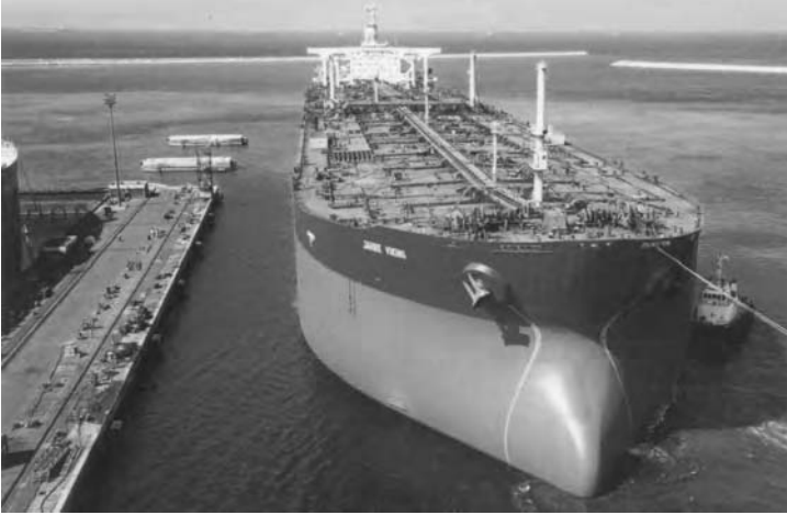
Fig. 5.2 Tanker structure. The ‘Jahre Viking’ at 564 000 dwt is the largest man-made transport in the world. It is seen manoeuvring with tugs off the Dubai Dry Dock. The size and sophistication of the modern tanker has changed considerably over the decades. World economics have influenced the capacity, while legislation has changed all future construction into the double-hull category. This vessel has recently been converted to a floating oil storage unit to prolong its active life.
