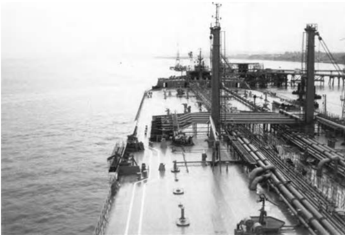
Fig. 5.10 Manifold and pipeline connections. Upper deck of an oil tanker showing the manifold, Samson Posts positioned to Port and Starboard, fitted with 5-tonne safe working load (SWL) derricks for lifting hoses to manifold connections.
