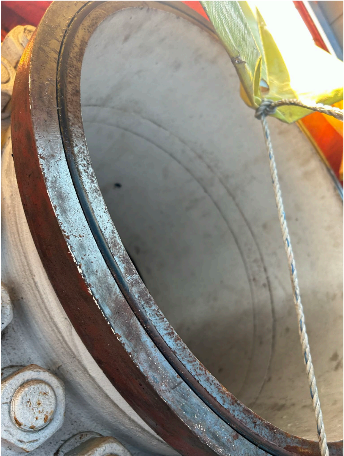
HRC Trunking and sealing face
