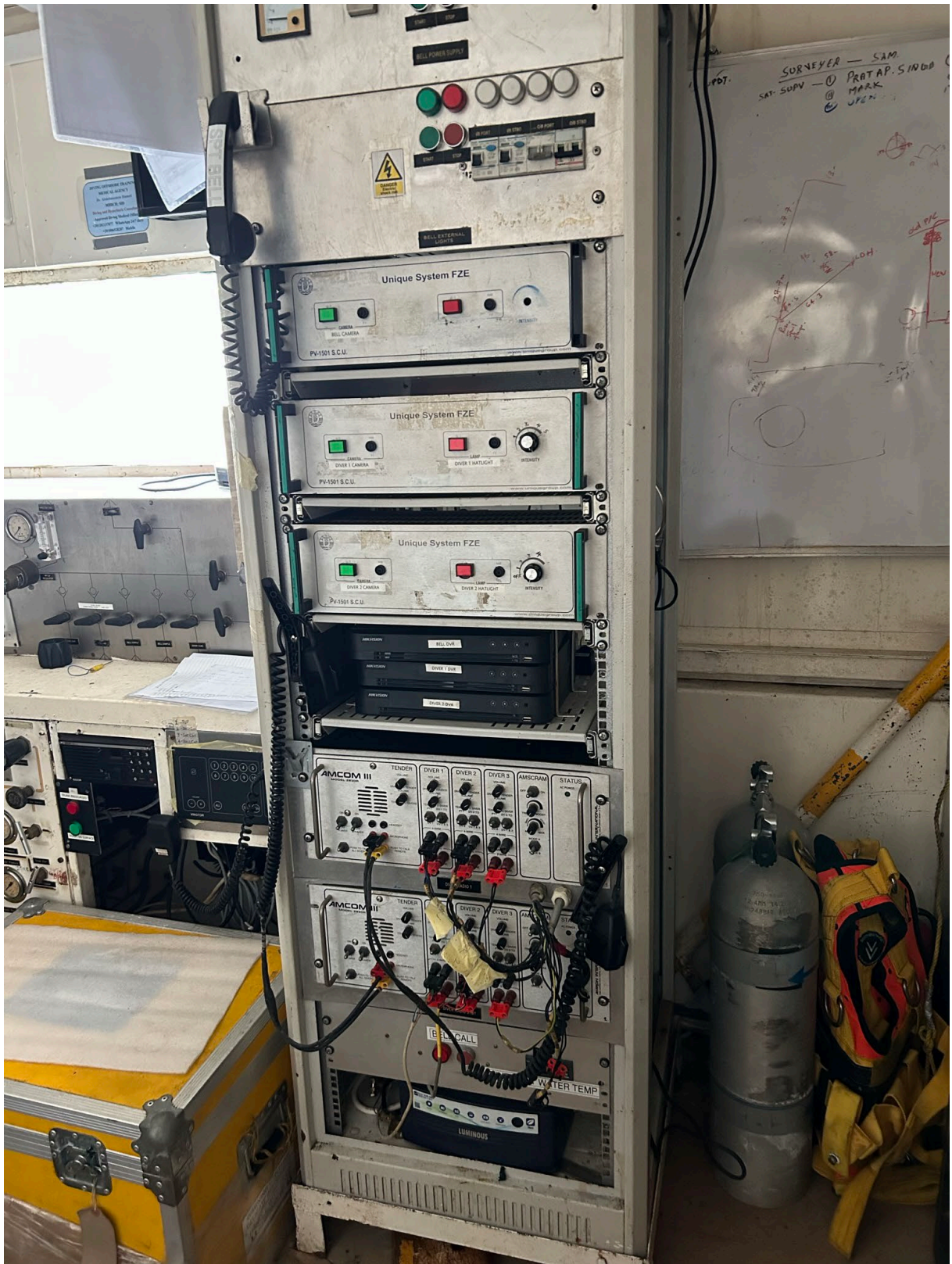
Saturation Dive Control Comms and Recording Uni
