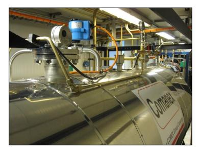
The manual switching manifold is provide to allow easy reconfiguration of the system.
