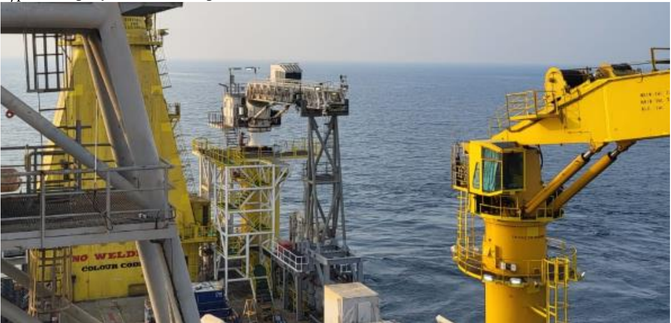
Typical Gangway installed on large Construction vessel
