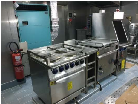
Galley (A deck)
