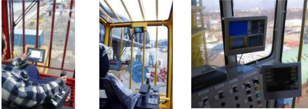
Figure 3: Operators cabin (typical)
