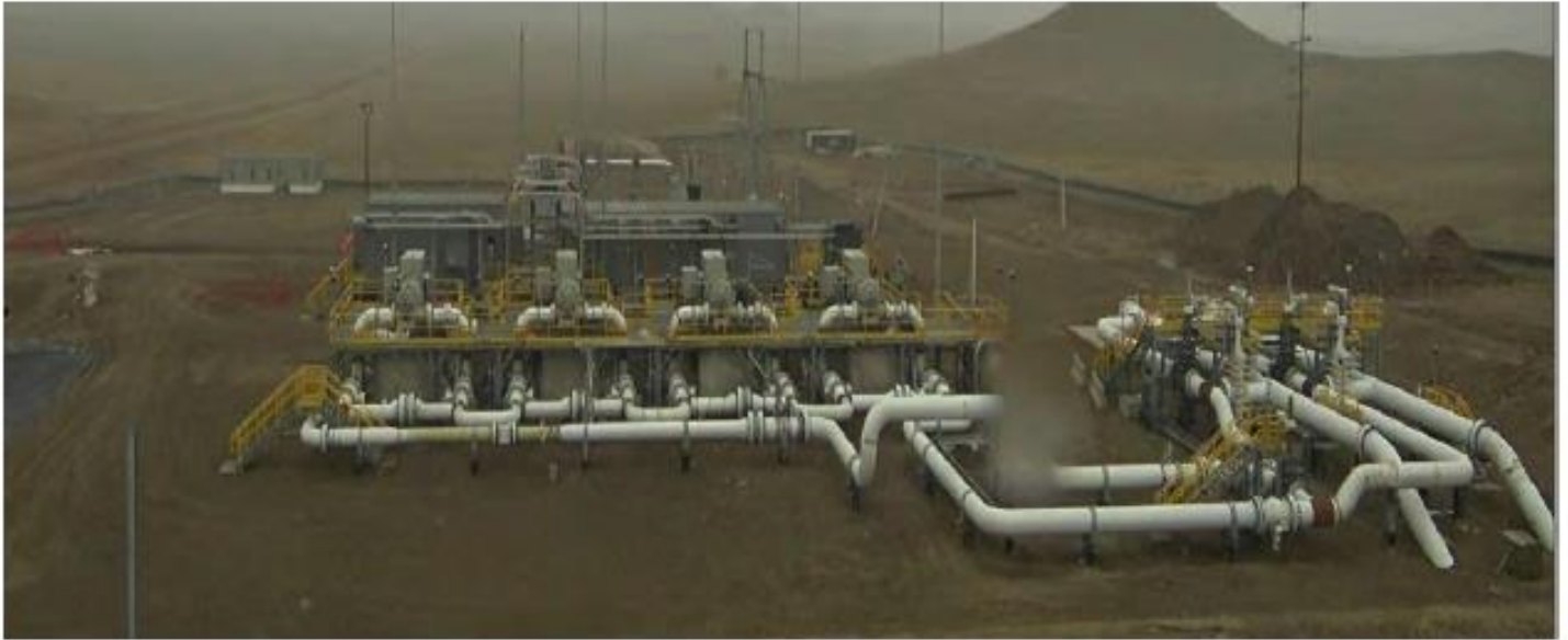
PUMP STATION 14 – 12 th April 2021
