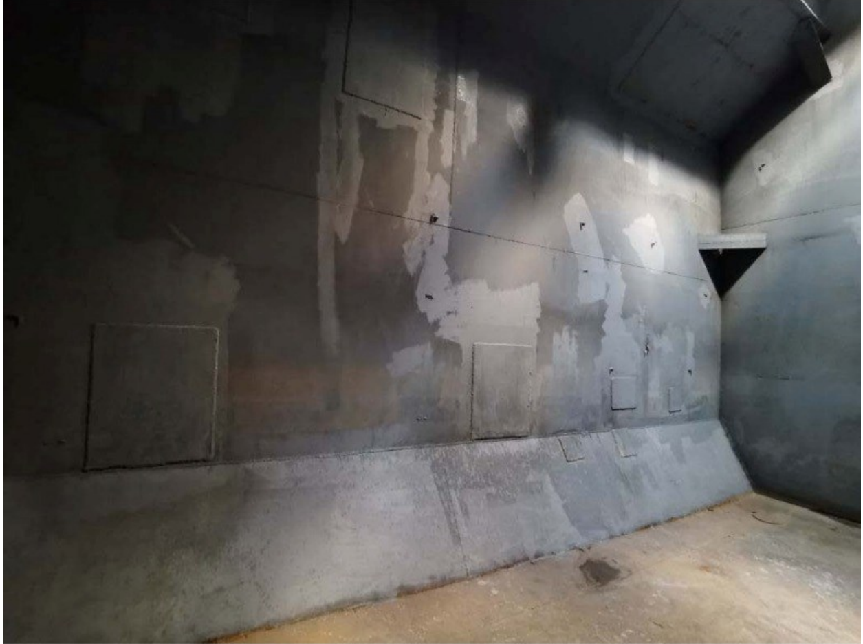
(64) Condition of No.2 cargo tank (S)
