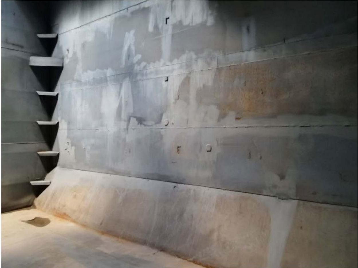
(72) Condition of No.3 cargo tank (P)
