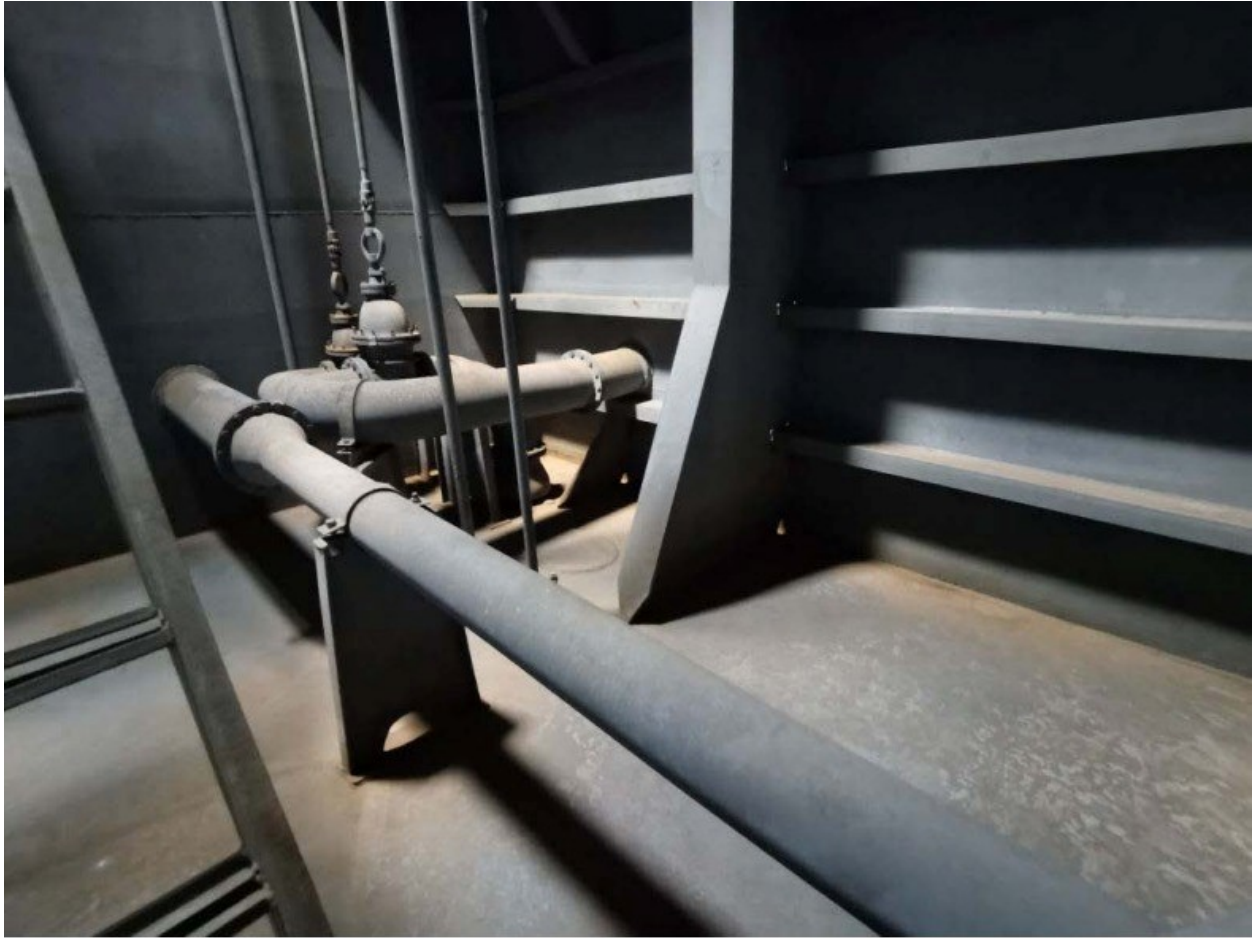
(50) Condition of No.1 cargo tank (S)
