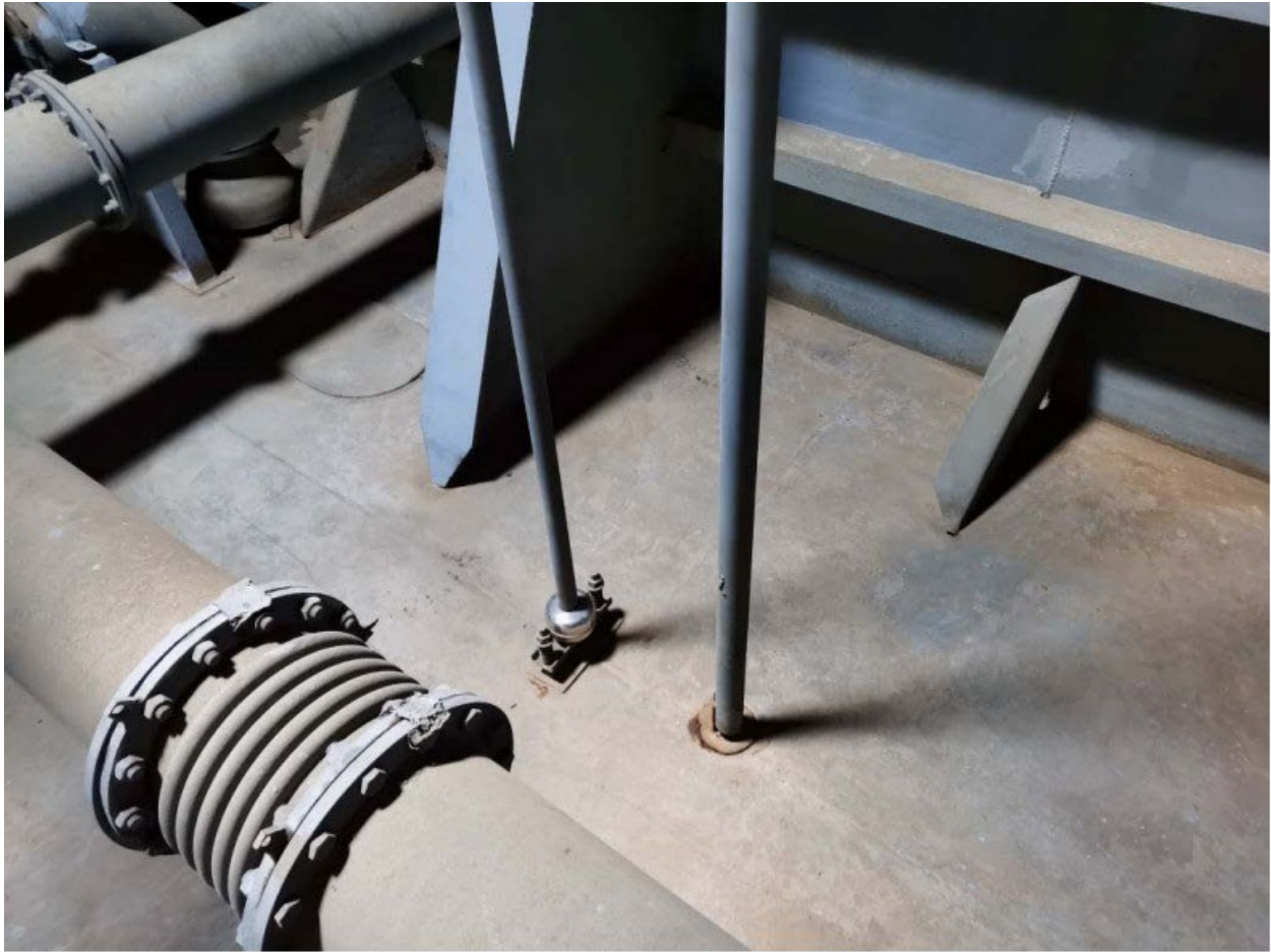
(68) Condition of No.2 cargo tank (S)
