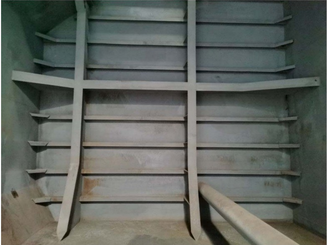
(69) Condition of No.3 cargo tank (P)
