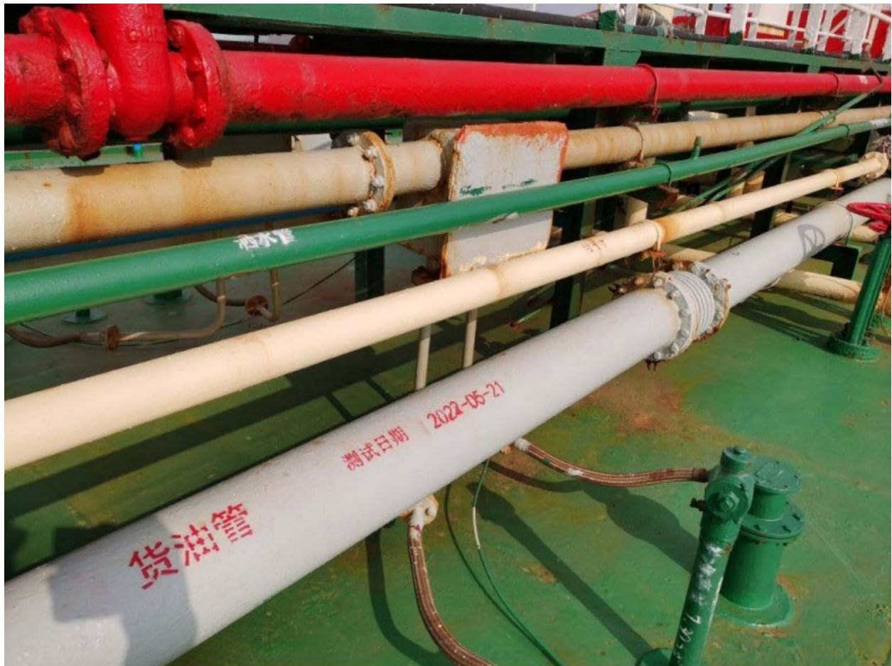
(32) Condition of pipe lines
