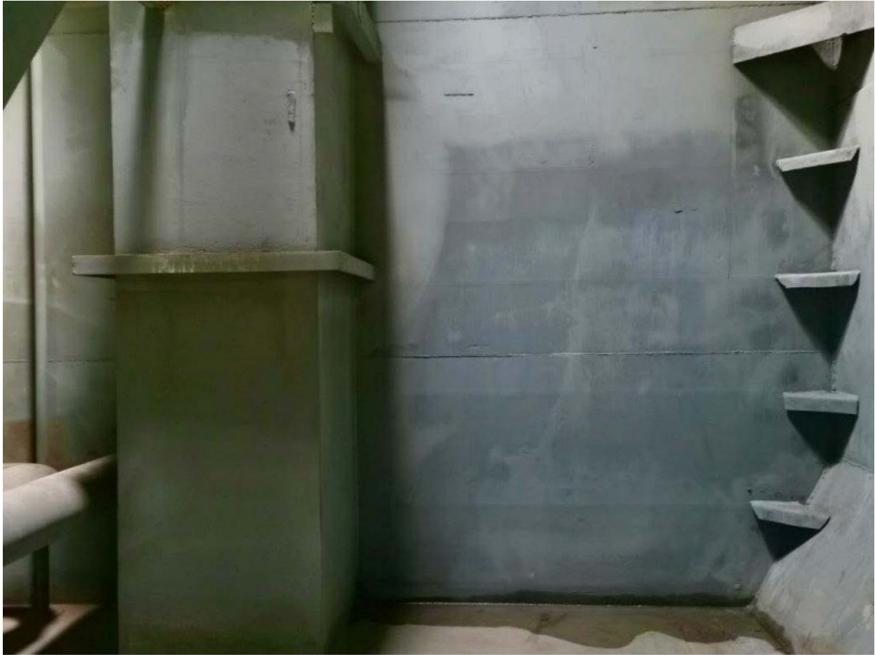
(56) Condition of No.2 cargo tank (P)
