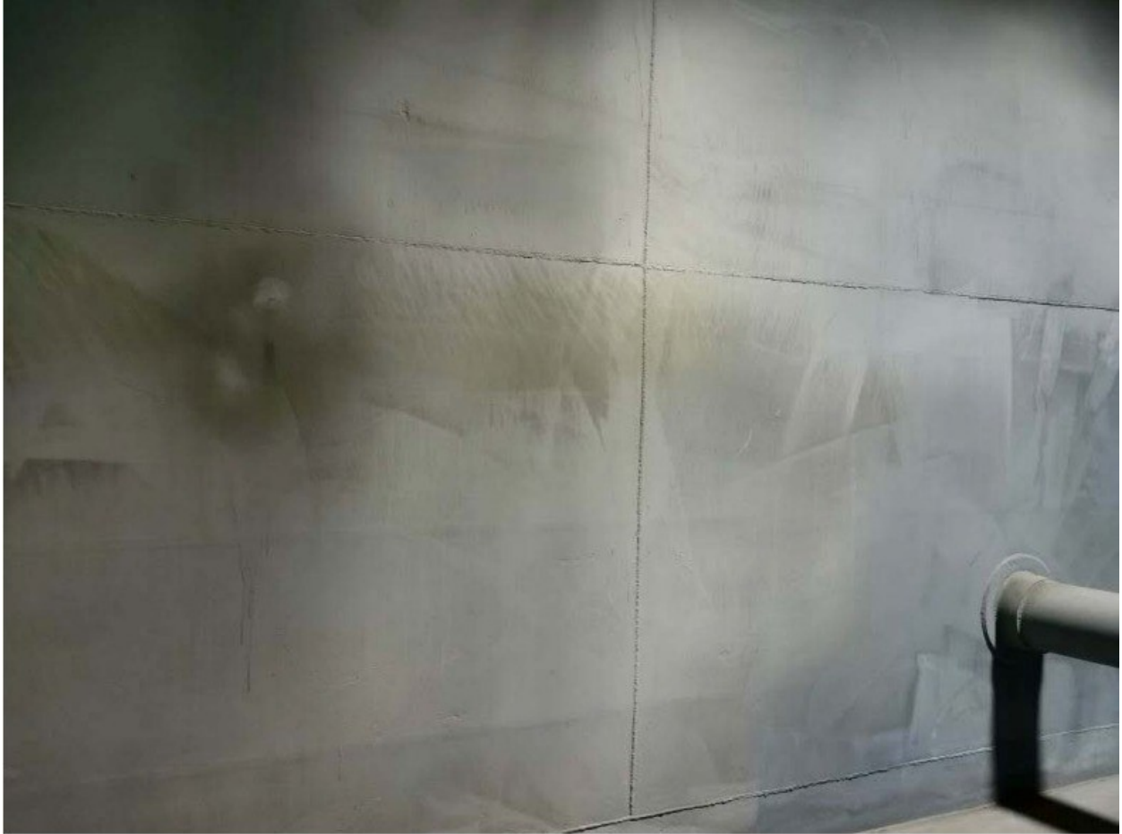
(58) Condition of No.2 cargo tank (P)
