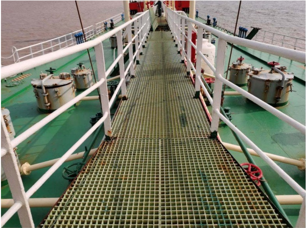
(29) The condition of catwalk
