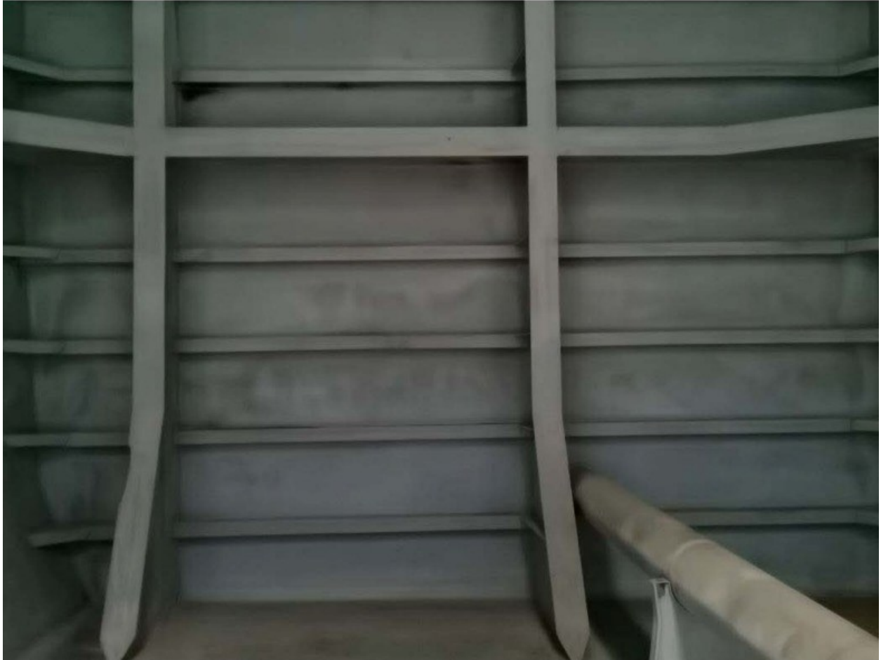
(55) Condition of No.2 cargo tank (P)
