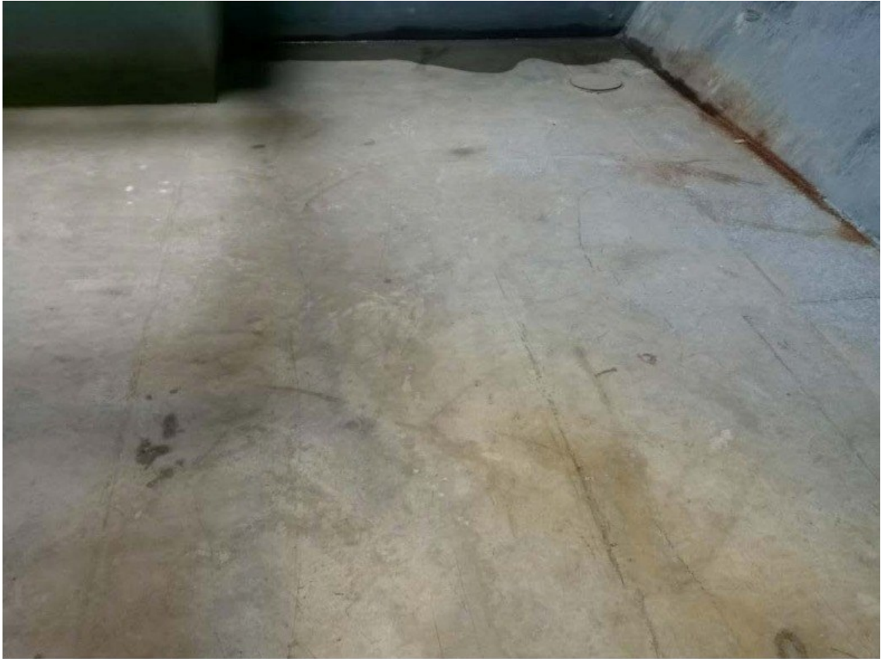
(60) Condition of No.2 cargo tank (P)
