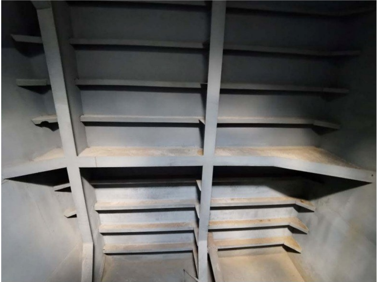
(39) Condition of No.1 cargo tank (P)
