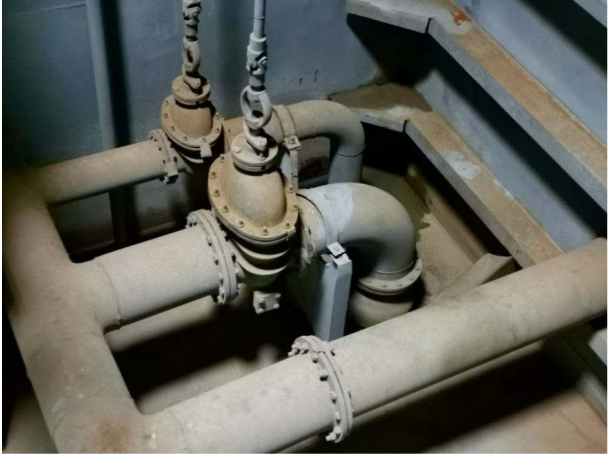
(67) Condition of No.2 cargo tank (S)
