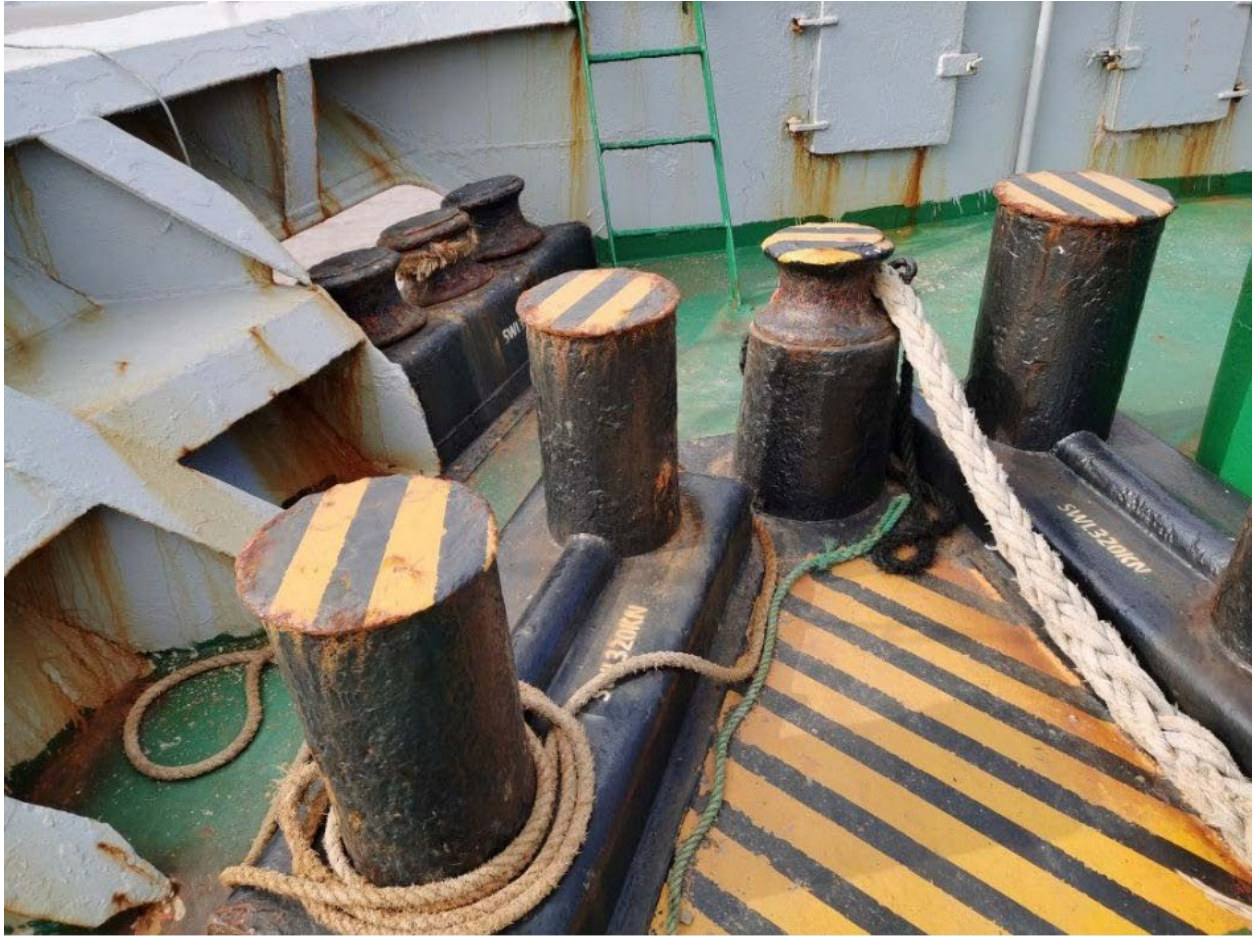
(18) Condition of mooring bitts, fairlead rollers
