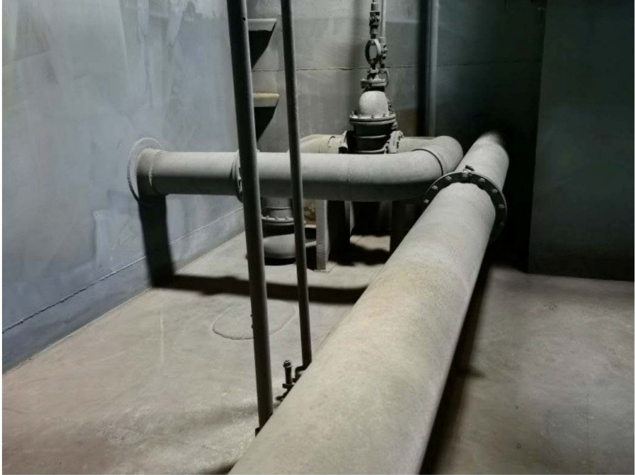
(59) Condition of No.2 cargo tank (P)
