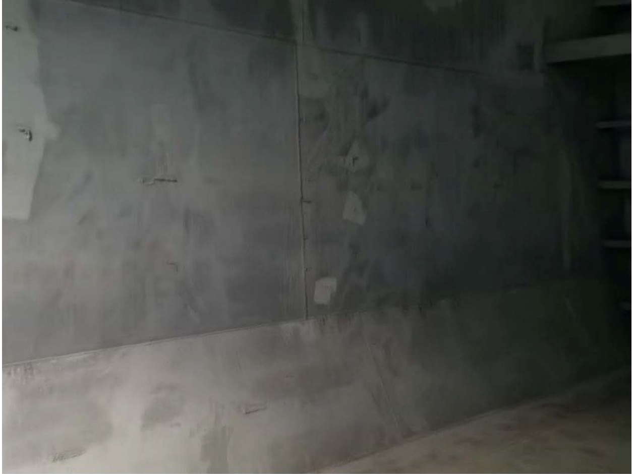
(57) Condition of No.2 cargo tank (P)
