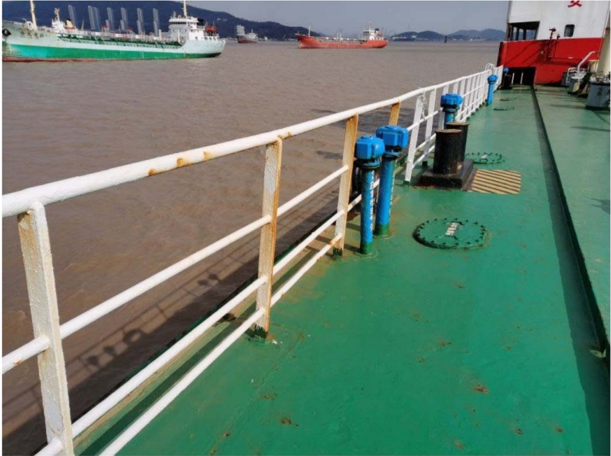
(25) Condition of main deck
