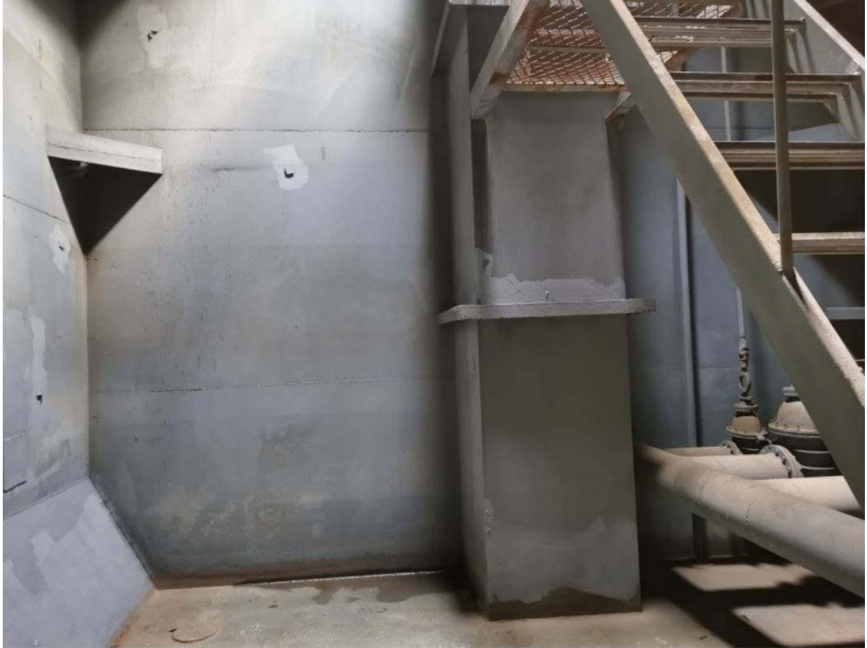
(63) Condition of No.2 cargo tank (S)
