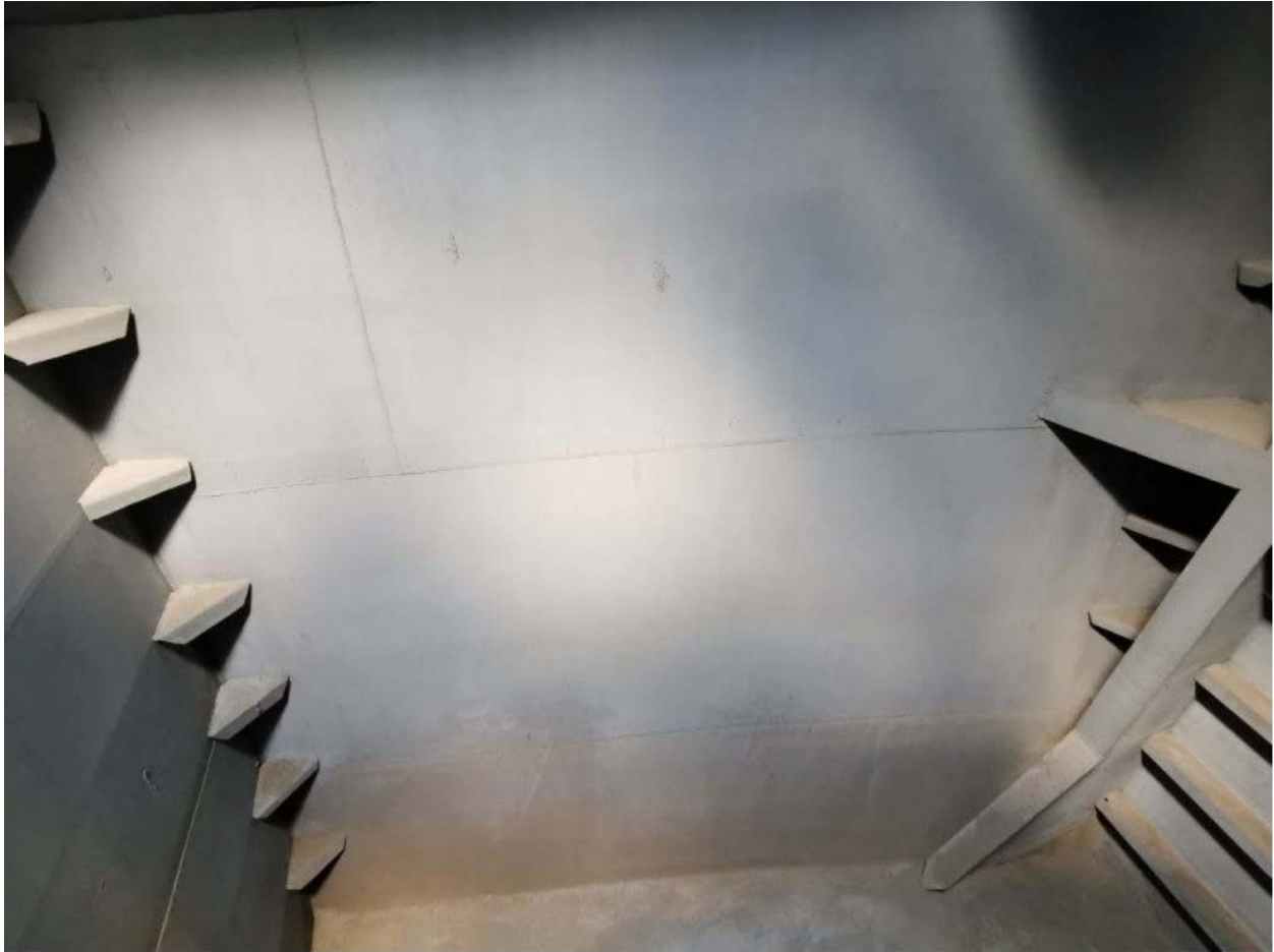
(40) Condition of No.1 cargo tank (P)
