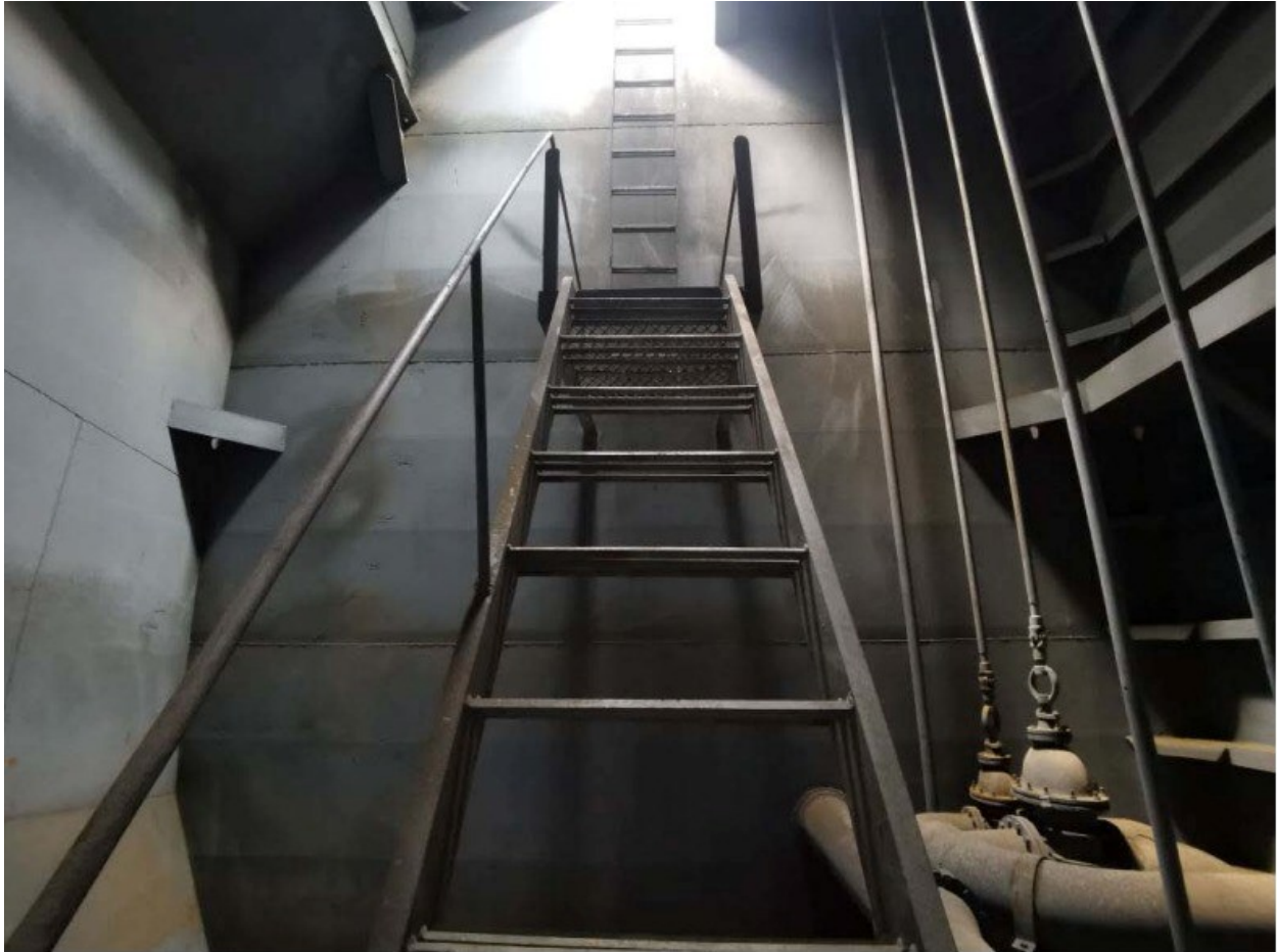
(51) Condition of No.1 cargo tank (S)
