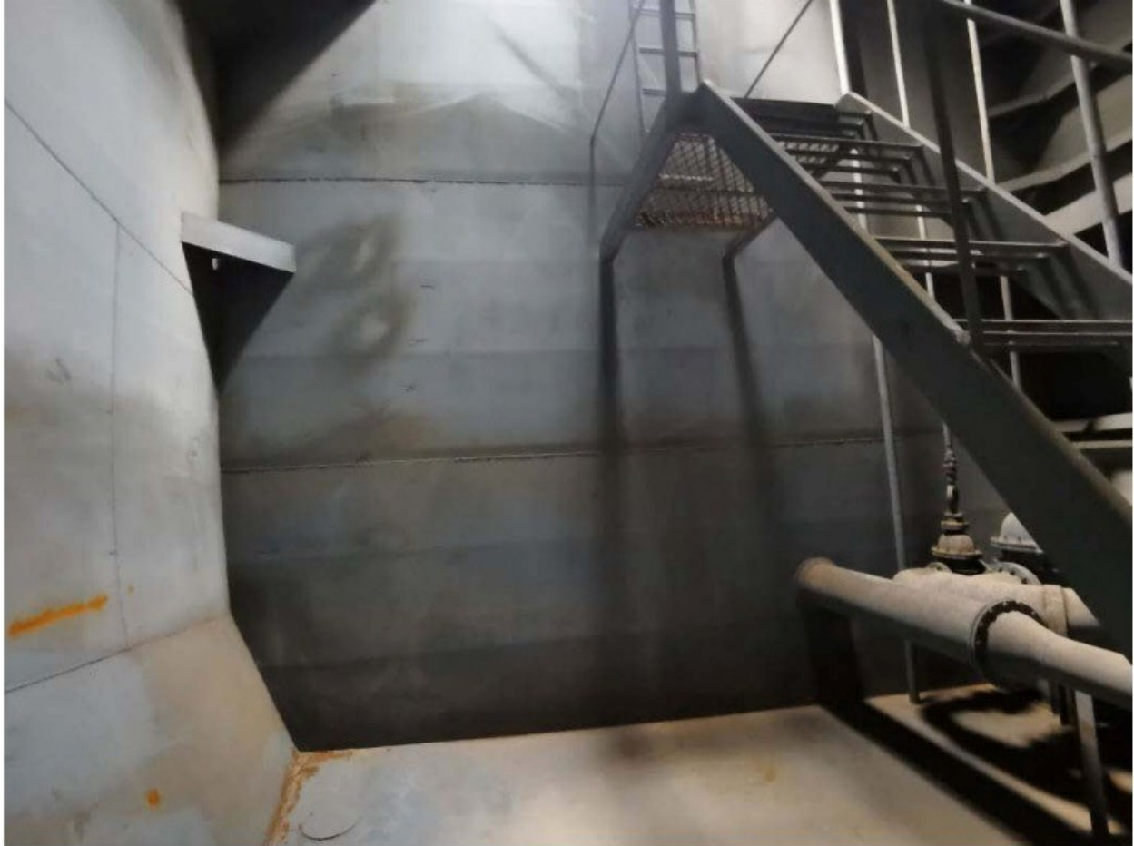
(47) Condition of No.1 cargo tank (S)
