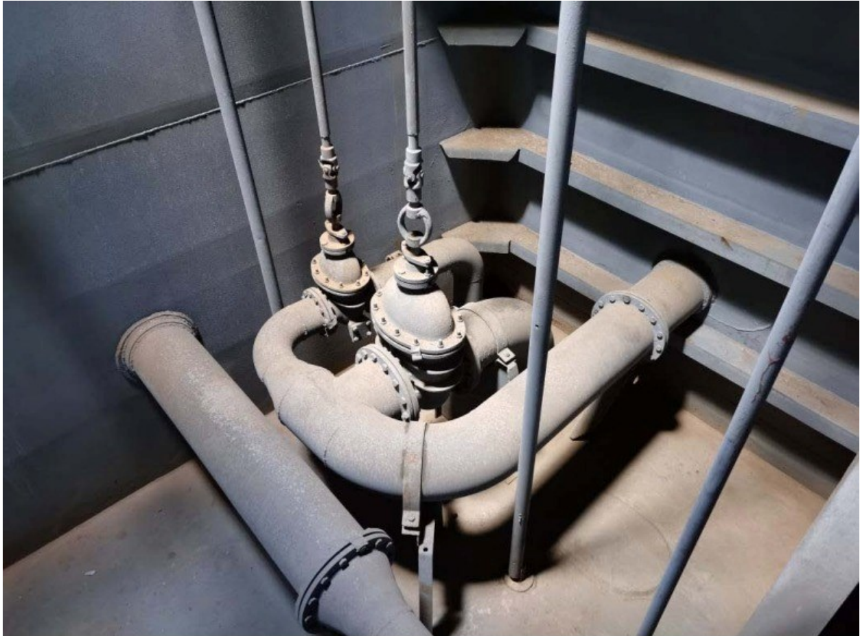
(52) Condition of No.1 cargo tank (S)
