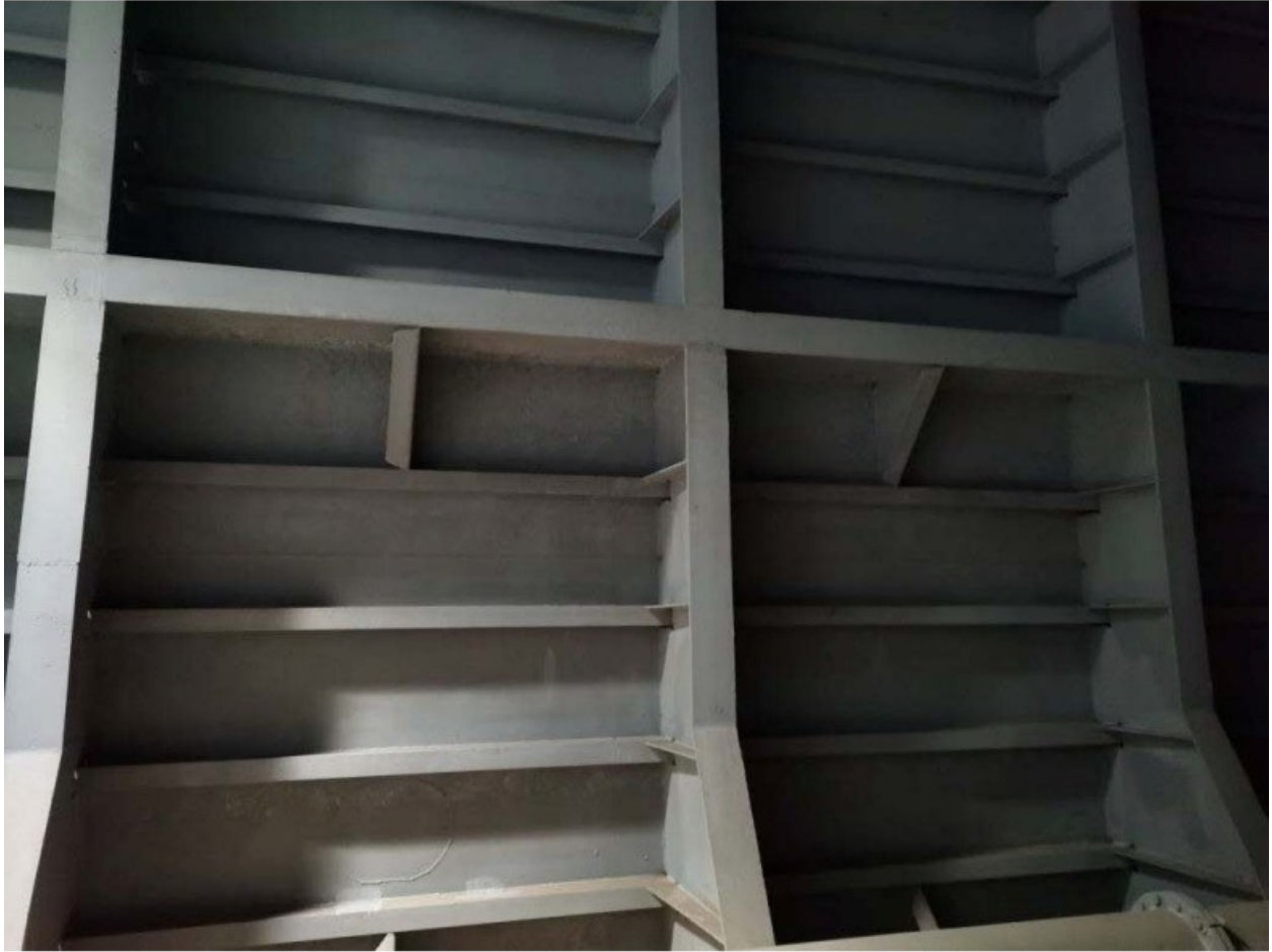
(65) Condition of No.2 cargo tank (S)
