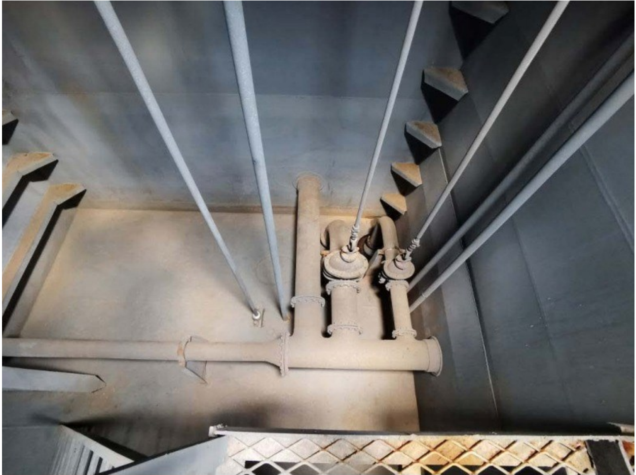
(42) Condition of No.1 cargo tank (P)
