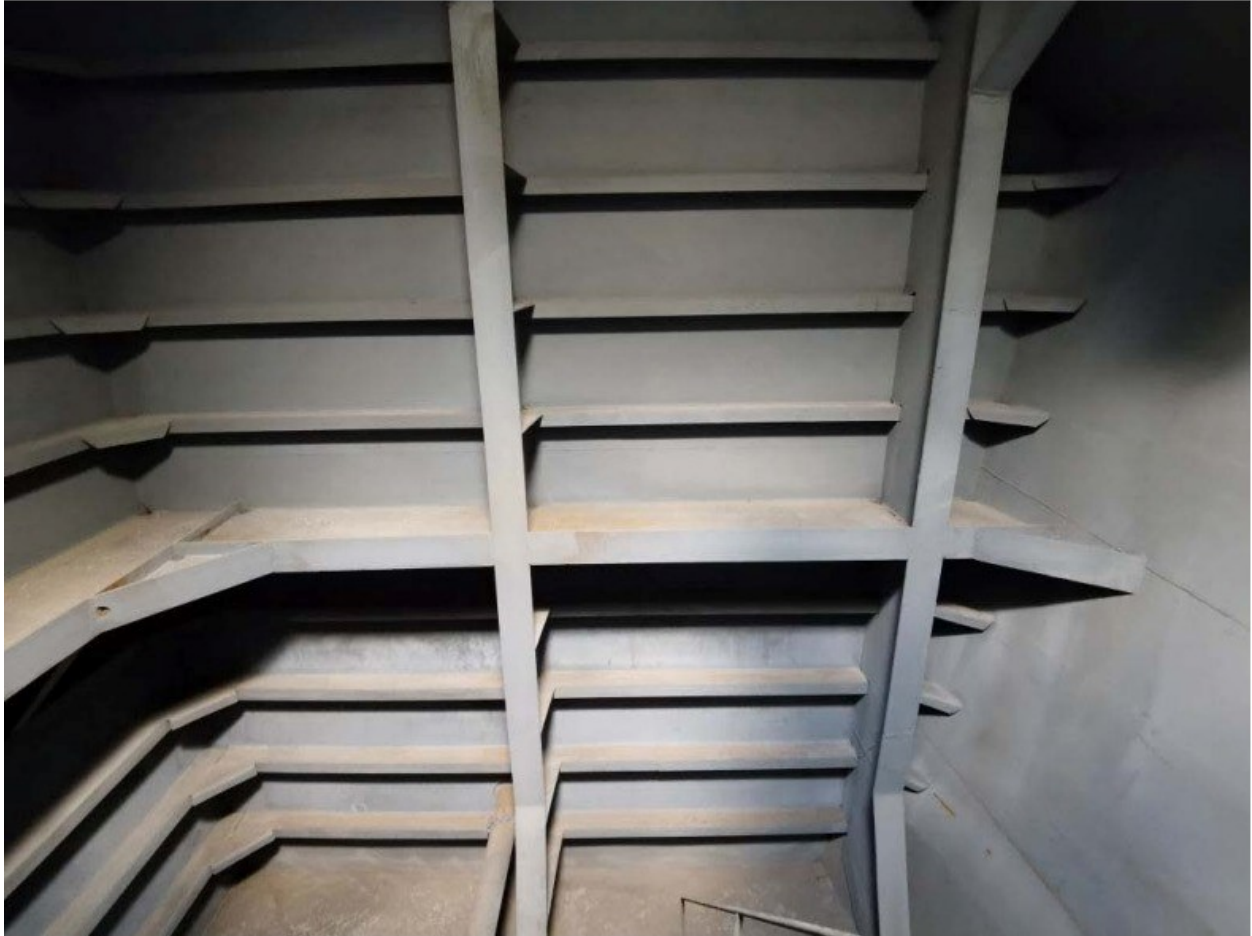
(46) Condition of No.1 cargo tank (S)
