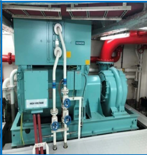
Pump Room-FIFI Pumps and Starters
